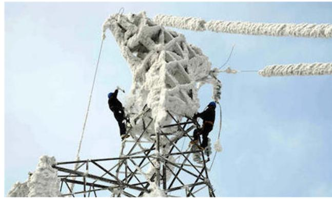
Fig. 15 Icing of transmission lines.
